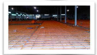
Over 33 kilometres of hot water piping efficiently heat the bus storage and maintenance areas
